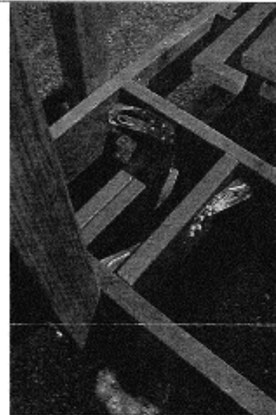
Guardrail-Post Connection
